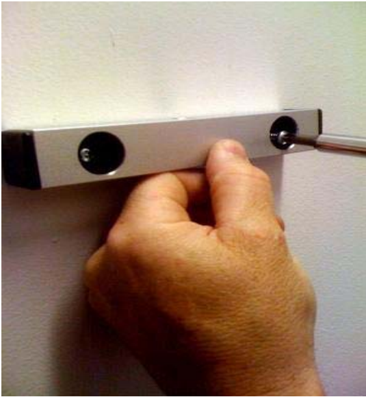
Fasten brace to the wall
